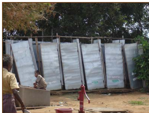
Toilets in the temporary shelter complex
