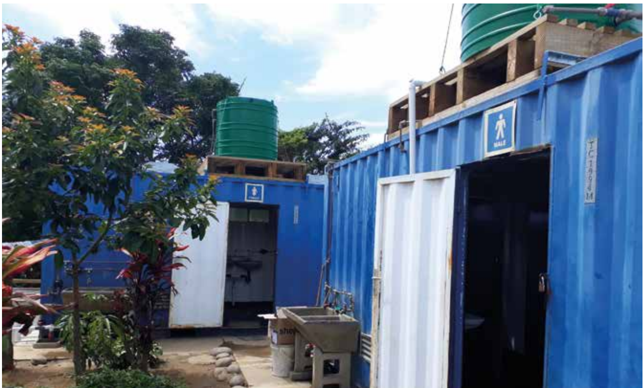
Figure 6: Community toilets in Durban, South Africa.
