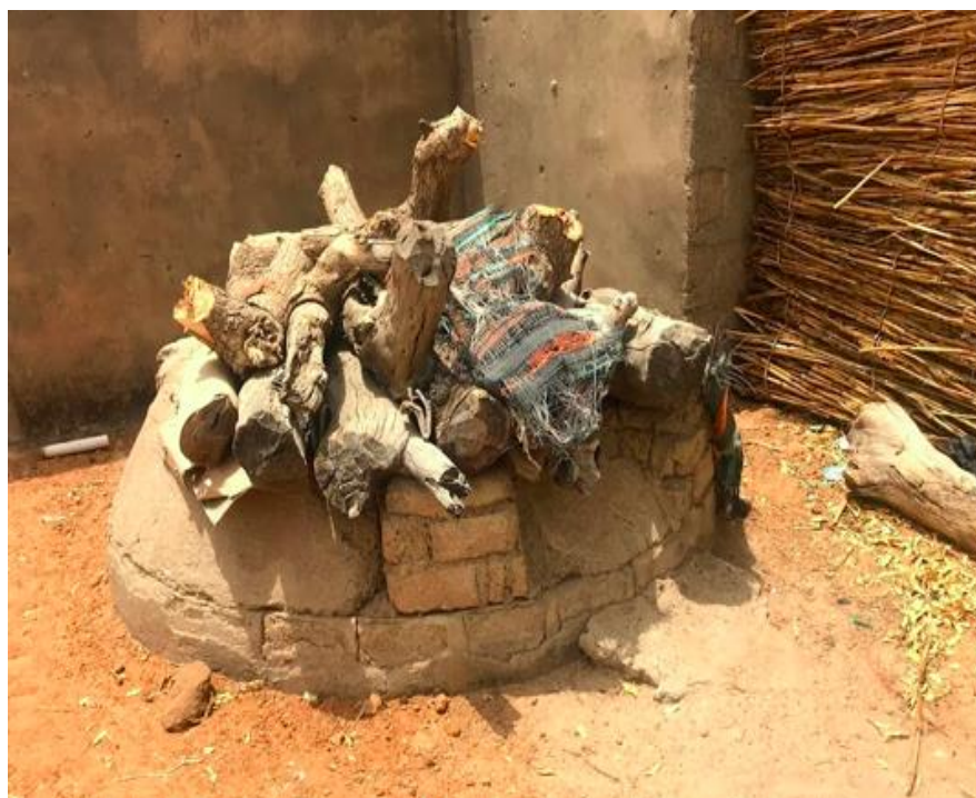
Figure 23: Open well in Yobe
