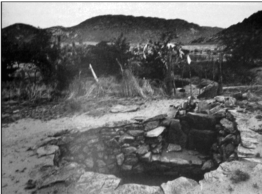
Illustration 1. A typical shallow pit well in South Africa, showing the platform from which the water was drawn.
